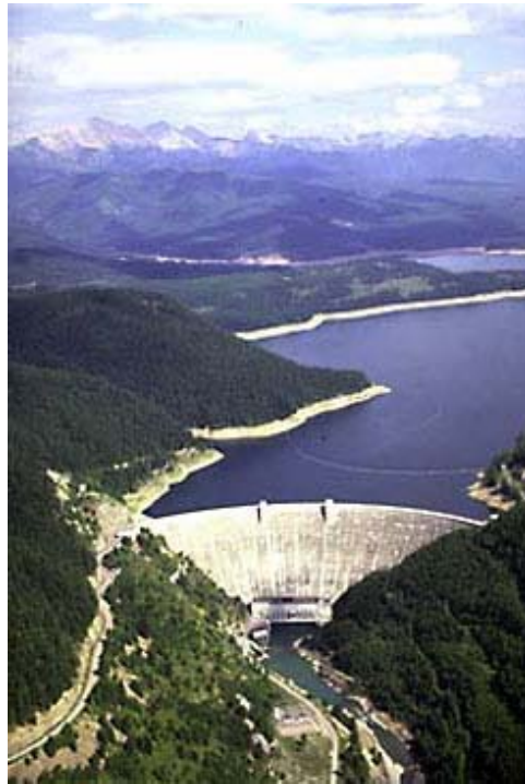
Figure 1-2 Hungry Horse Dam built with fly ash concrete in Montana, USA ( http://www.usbr.gov/dataweb/dams/mt00565.htm )
